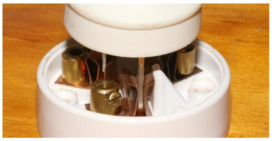
This plug was easily inserted without the lid to guide it into place, all but impossible with the 'new style board'
